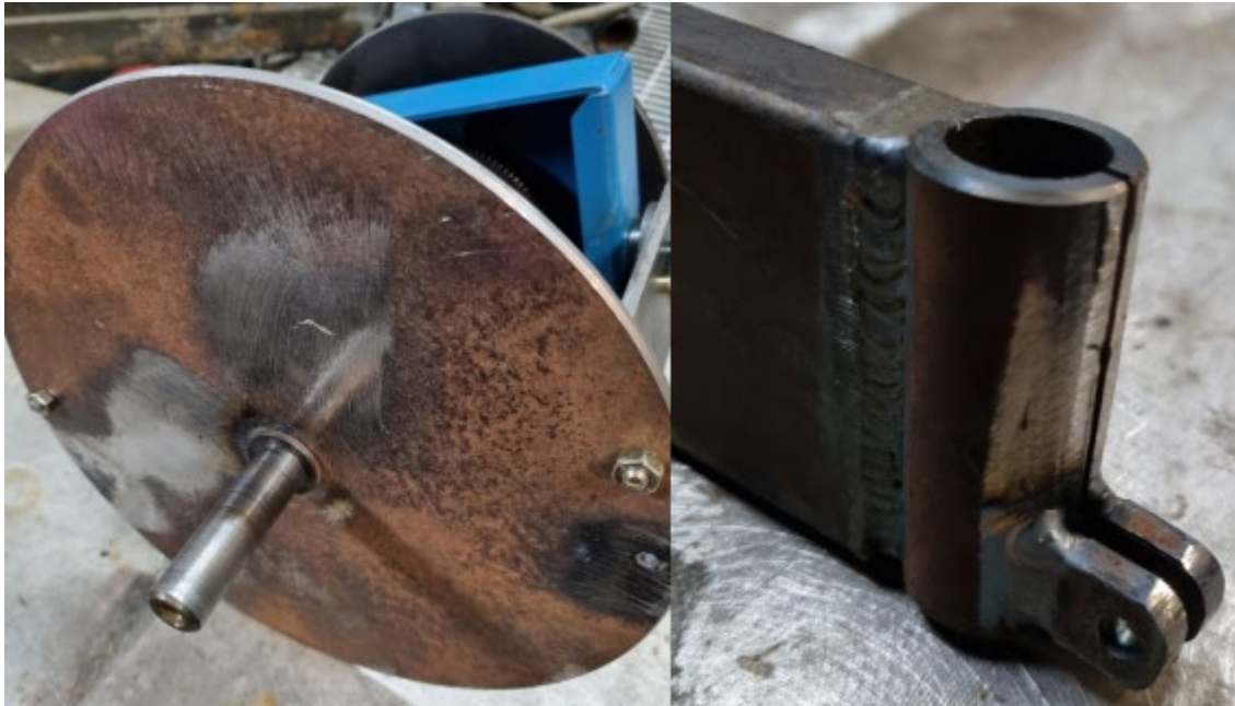
Fig. 35. Welding the pin into the bushing plate and of the sleeve into the turntable arm
