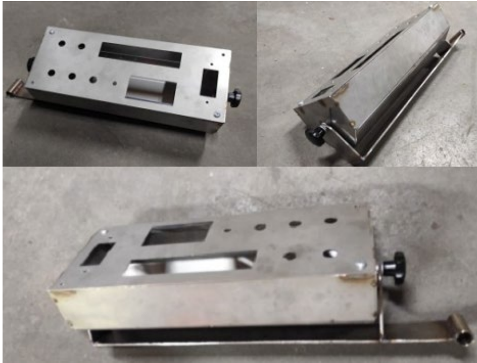
Fig. 46. Welding and assembly of the control panel support structure
