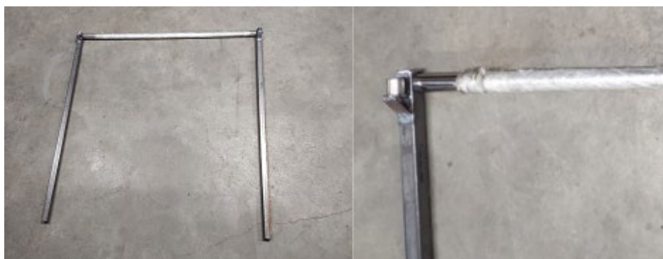
Fig. 48. Construction of a protective screen frame made of 30x30x2 steel profiles
